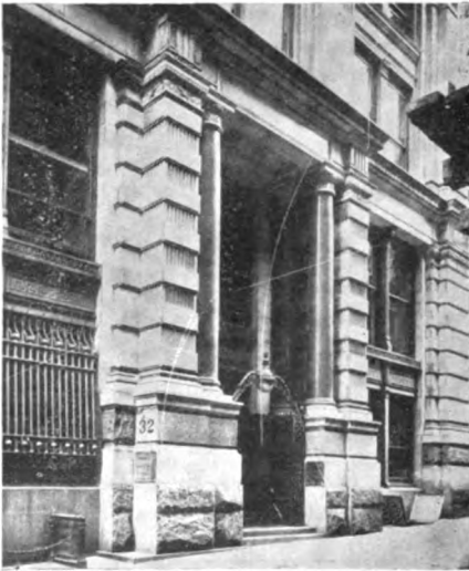
Liberty Street Entrance to Main Office.
